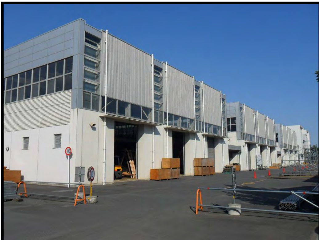
B Building ( Department of Building )
